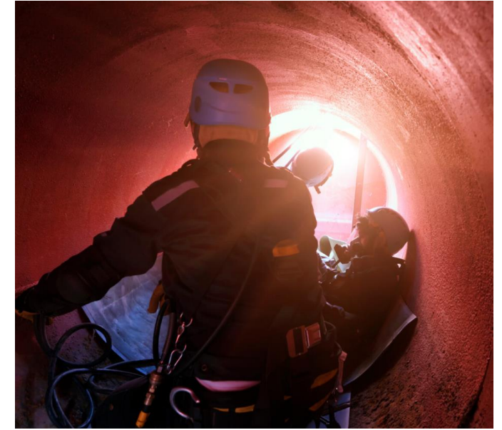
Fig 1 Difficult working condition
