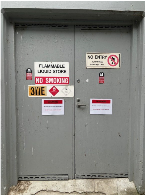
Dangerous Goods Store Door
