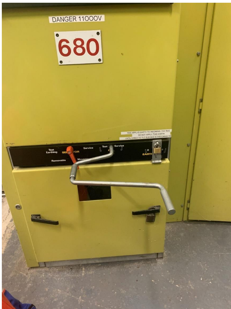
Temporary warning label applied to the switchboard earthing handle insertion point
