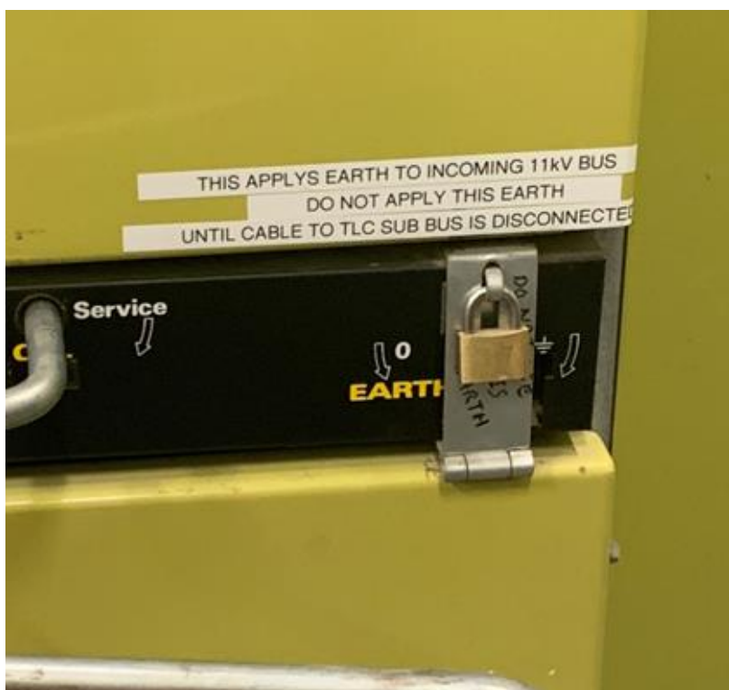
Temporary warning label applied to the switchboard earthing handle insertion point
