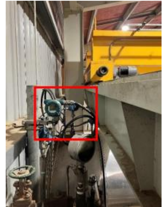
Contractor's work position, in relation to crane
