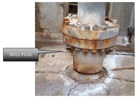
During clean up of the wellhead after a the well had been abandoned, one of these bull plugs fell off due to indirect shock loading from hammering on the CHF. If the well had been in service, this would have led to a loss of well containment and serious risk to any personnel on the cellar.
