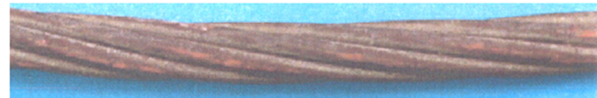
(a) Light Visual Damage – Light Weathering
